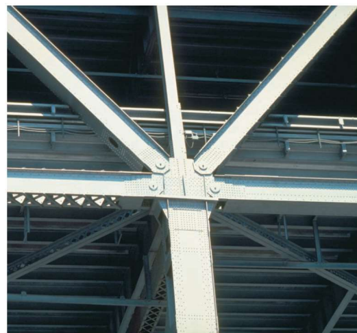
Bridge with pin-joints.
